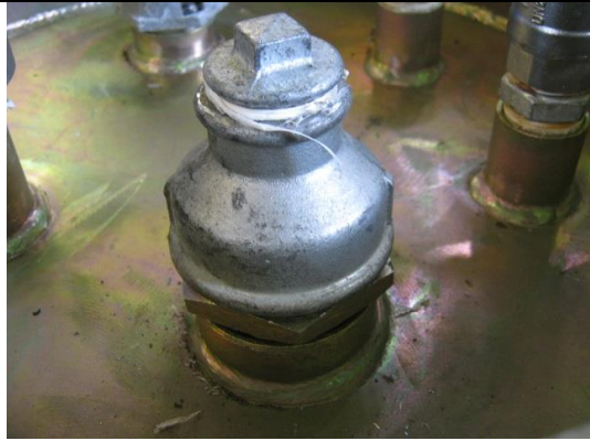
Filling line connected to 2" BSP overfill prevention valve
