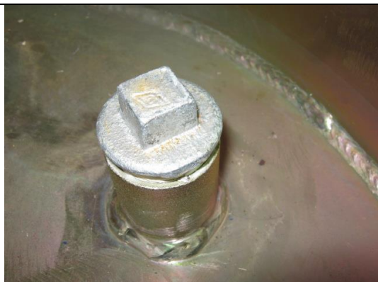
Spare suction line within manway enclosure
