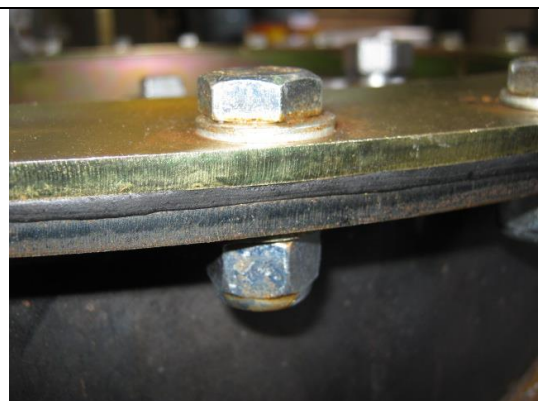
Rubber gasket sandwiched between flanges
