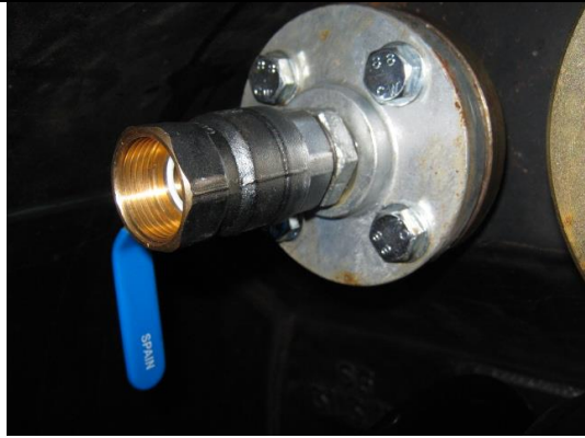
Suction line, located LHS of bulk head
